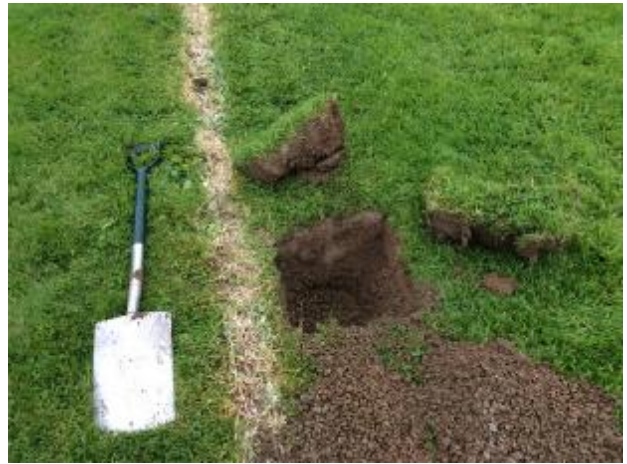
Figure 8: The main drain was dug and the aggregate. There was a layer of 100mm of topsoil over the aggregate which was found to be significantly blocked with soil in the upper 100mm. Below this the aggregate was cleaner.
