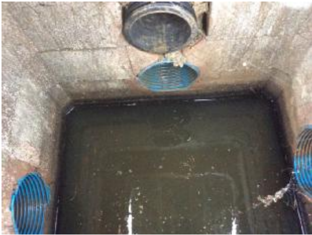
Figure 7: The North western pitch side manhole was loose and damaged. It was lifted slightly to allow a photograph to be taken. There were a number of inlets and outfall. There was only one in a west direction that showed an evidence of water flow. The middle south pipe was investigated in figure 8.
