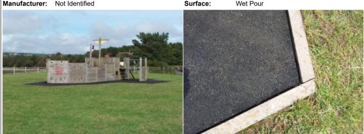
**Finding:** There are gaps opening between the surfacing and **Action:** Monitor for any further deterioration and repair as the edging surround or between the joints in the surfacing required
