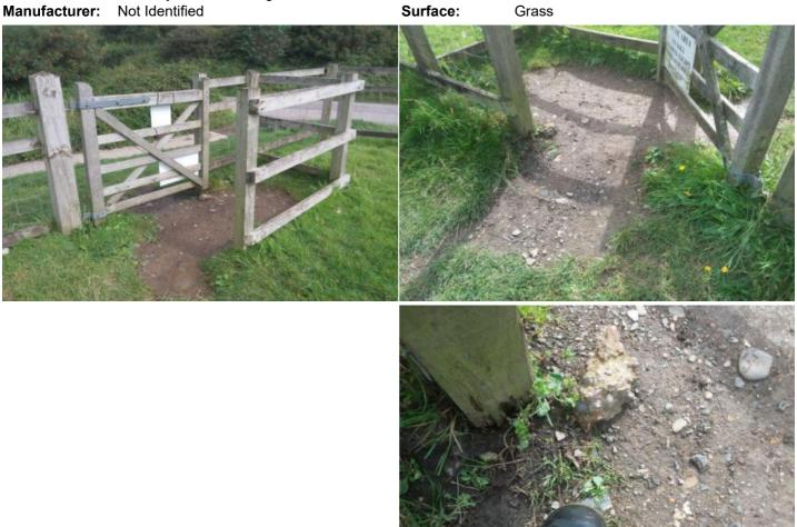
**Finding:** The area under the gate has eroded leaving uneven areas, or the concrete foundations exposed, resulting in trip hazards at the entrance/exit to the playground
