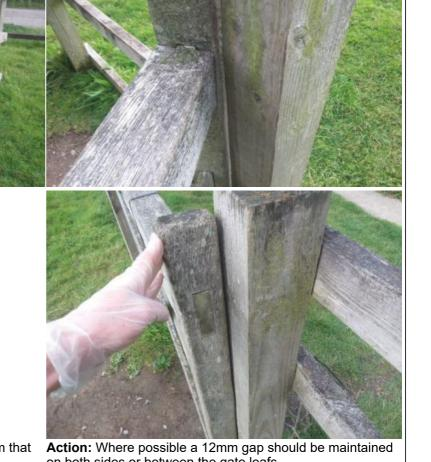
**Finding:** There are openings that are less than 12mm that could trap or crush fingers
