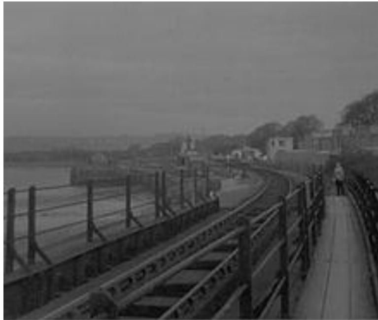
Fremington station and quay in 1970 shortly after the steam cranes were removed
