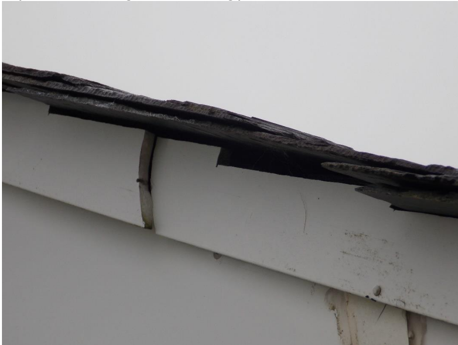
Gaps at the western gable end offering potential bat access
