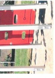
elevates the posts 20mm from ground level to galvanised steel footings. The steel footings The main tower posts of either pine wood or aluminium are all equipped with hotdip avoid contact with surfacing material.
